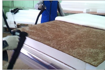
Manual spray application
